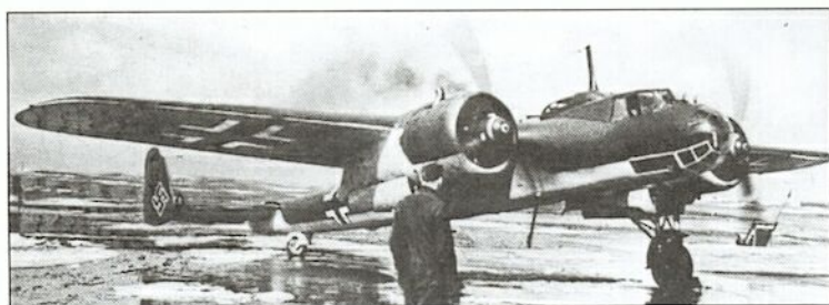
Above: The Do 17P-1 still equipped many reconnaissance units on the outbreak of war, and the similar Do 17M-1 bomber was also on charge. Note the slim fuselage of these early aircraft.
