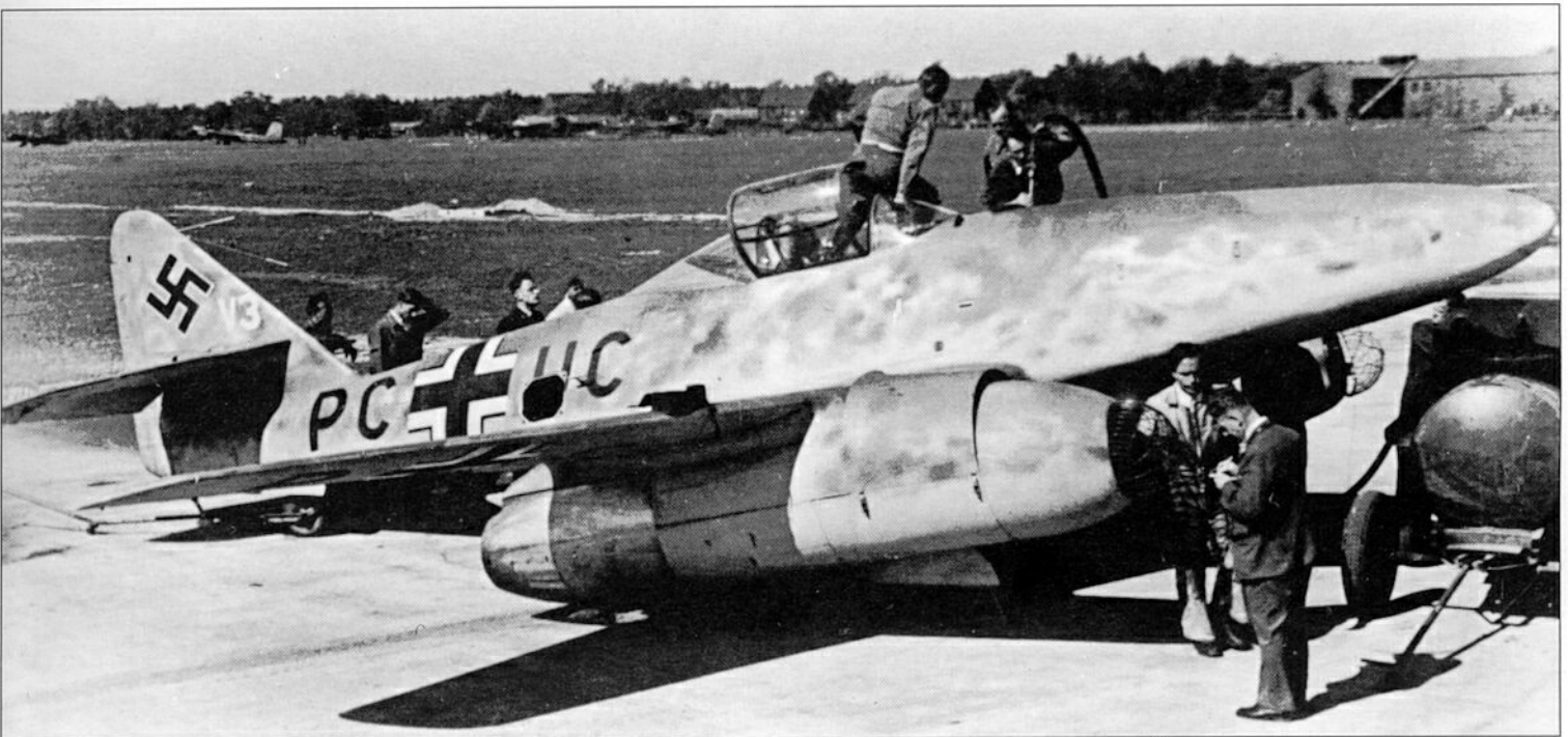
Above: A female Luftwaffe auxiliary signals to the pilot of an EKdo 262 or EJG-2 Me 262A-1a. In the intercept role, the Me 262 could carry 24 underwing R4M rockets in addition to its built-in armament of four 30-mm MK 108 cannon. The aircraft had 100 rounds for each of the upper guns, and 80 for each of the lower pair.
