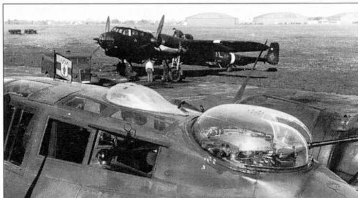
Below: The combination of the dorsal turret and lateral-firing weapons gave a good field of fire, but all were operated by just the radio operator.
