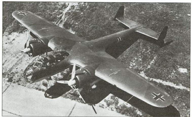
Illustrating the broad slab wing of the Do 17 is this early Z-1, the first bomber variant with a redesigned cabin. This version was markedly underpowered and had a reduced bomb load to compensate.
