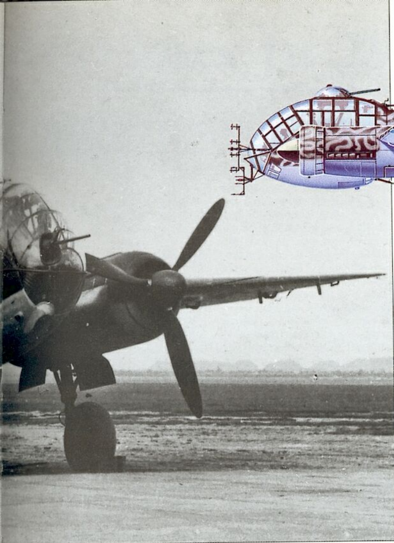
FuG 200 Hohentwiel-equipped Ju 188D-2 of 1.(F)/122 at Kirkenes, Norway in 1944.
